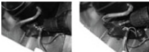
(2) Loosen two screws on comp base
